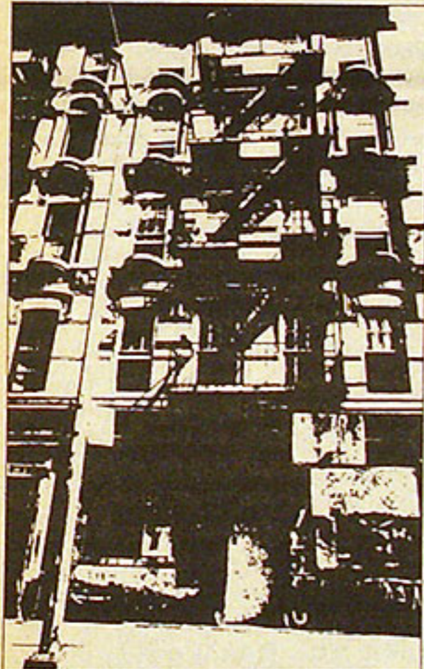
Decaying urban housing.
